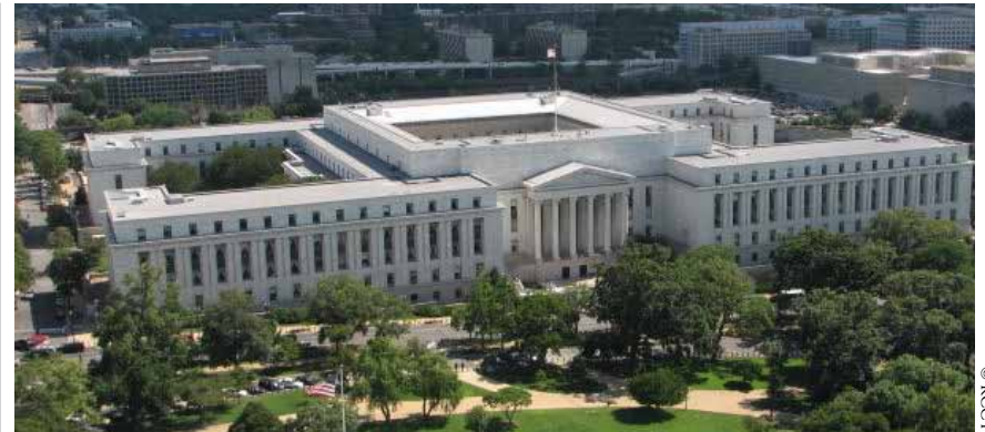
The Rayburn House Office Building BIPV (Building Integrated Photovoltaic) Roof
