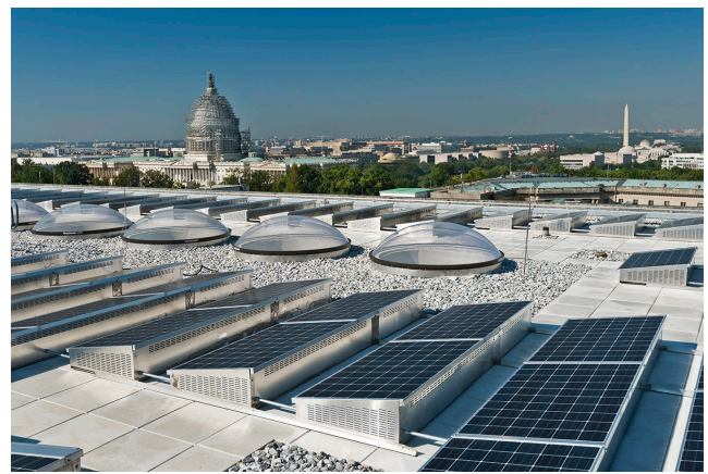
Hart Senate Office Building roof showing skylights and photovoltaic (PV) panels
